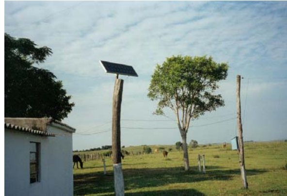
Solar Panel is connected to an electrifier that powers a 10 000 V fencing system
